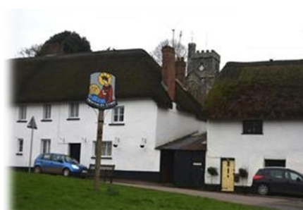
Box 11: Thatched Houses in Newton St Cyres Village
